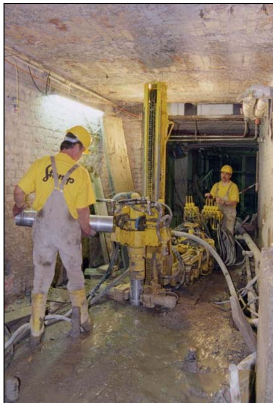
FIG. 6: Drilling operations for pile manufacture
