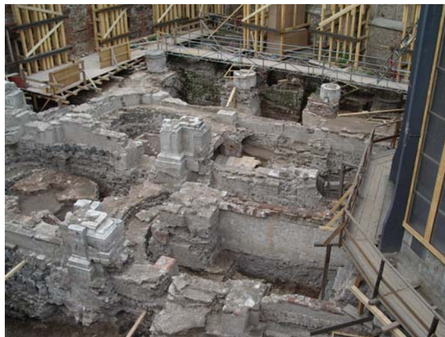
Fig. 15: Digging field surface
