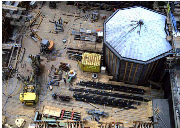
Fig. 16: Drilling work in the area of the digging field
