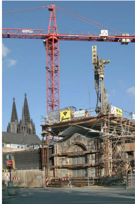
Fig. 13: Drilling work from working platform
